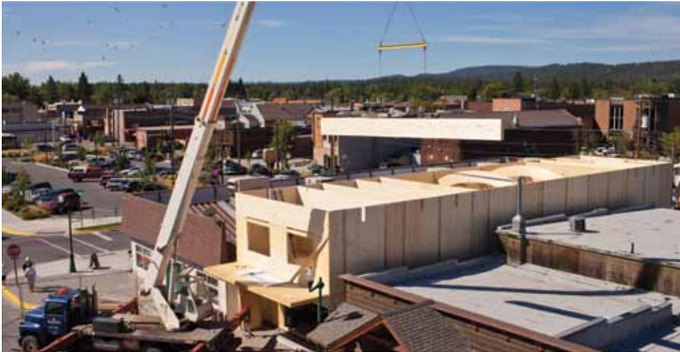
**Speed record:** Taking speed of construction to an entirely new level, the two-story Long Hall in Whitefish, Montana, designed by Datum Design Drafting and engineered by CLT Solutions, took just five days to erect and gave the owner a sustainable, energy-efficient building. It was the first commercial building in the U.S. made from CLT.
